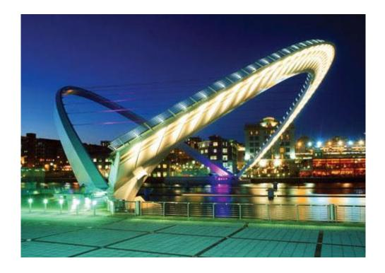
Millennium Bridge (2001), Gateshead, by architects Wilkinson Eyre and structural engineers Gifford The bridge pivots upwards to allow tall boats and ships to pass underneath
